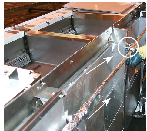
Figure 6. Rear cabinet connection holes. Note oil return line fittings.
